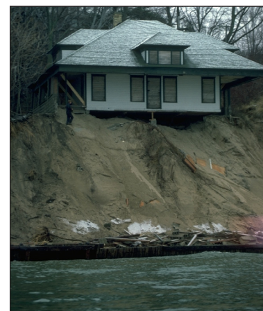
High lake levels on Lake Michigan in 1986 caused severe erosion. Photo: NOAA
