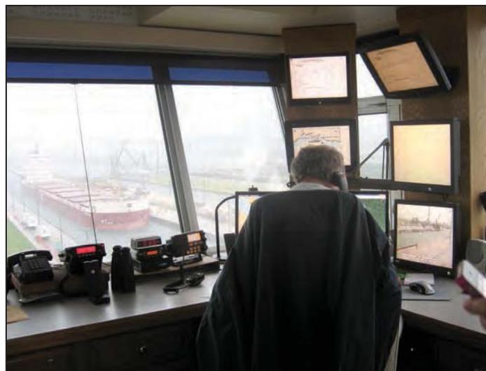
US Army Corps of Engineers lock master uses NOAA water level data to guide freighter traffic through the St. Marys River locks at Sault Ste. Marie, MI.
